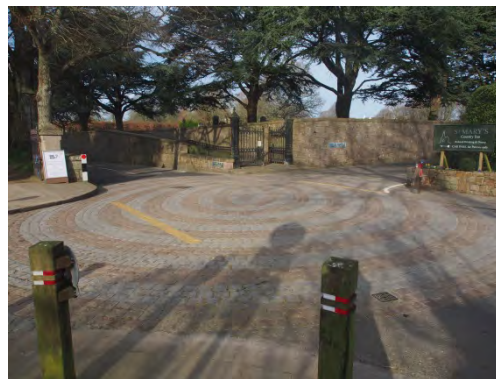
Granite sets used in St Mary's Village to create a traffic-calming feature which also contributes to local character and provides an attractive setting for the church and cemetery.
