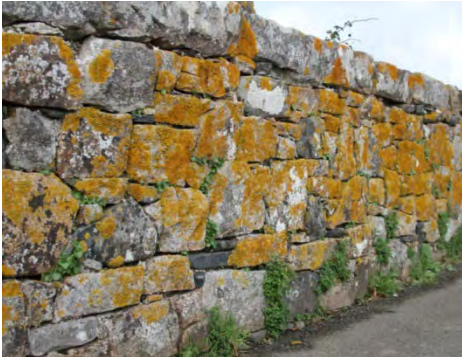
Random coursed stone wall with horizontal cope, St Aubin's Bay
