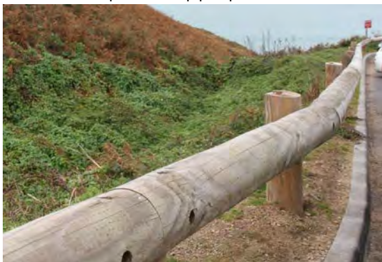
Chunky timber, reinforced with galvanised metal, provides a robust vehicle barrier that is appropriate for rural locations – though would integrate better without pre-cast concrete kerb
