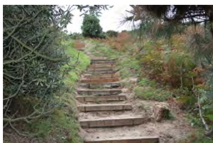
Chunky timber sleeper steps help control erosion on popular routes
