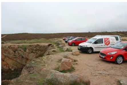
Boulders sourced locally make a low maintenance vehicle barrier, though would be better not set out in straight lines
