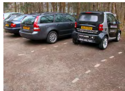
Salvaged granite setts used to demarcate parking spaces within crushed stone surfacing
